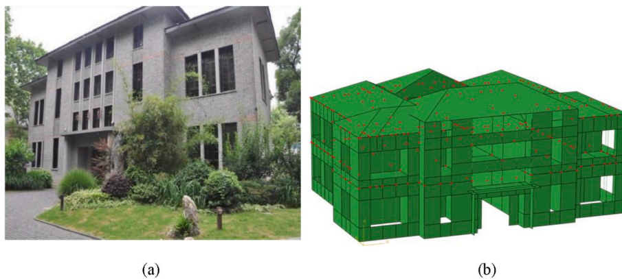
Fig. 9. The three-story reinforced concrete structure. (a) Shows the photo of the three-story reinforced concrete structure; (b) shows the finite element model of the three-story reinforced concrete structure and selected nodes.
